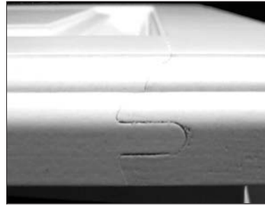
Example of end joint separation
